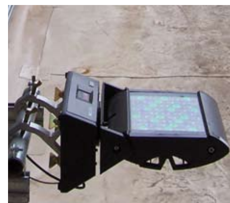
One of the 81 SGM Palco 3 LED color wash fixtures that uplight the Grant Hotel
