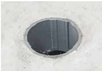
Cut box top level with concrete
