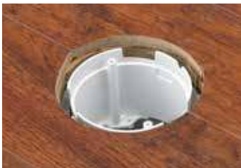
Install Adjustable Mounting Cup and level with finished flooring CFBS1R4CUI
